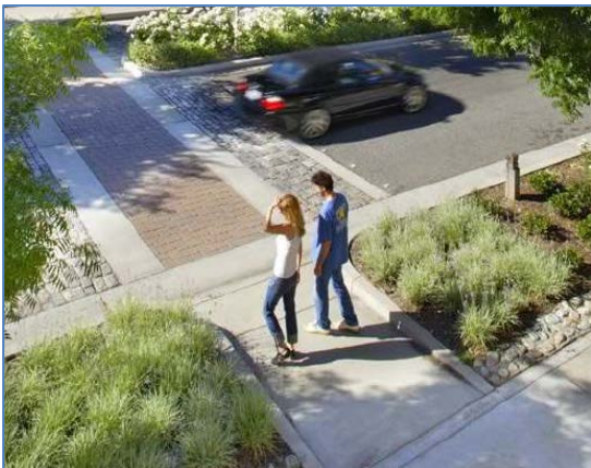
Figure 1.14 – Example of raised pedestrian crossing
